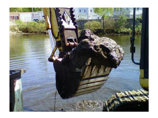
Gravity clamshell bucket on crane, good for softer sediments as down-force is bucket weight only, longer reach and swing possible, more difficult to monitor excavation depths
