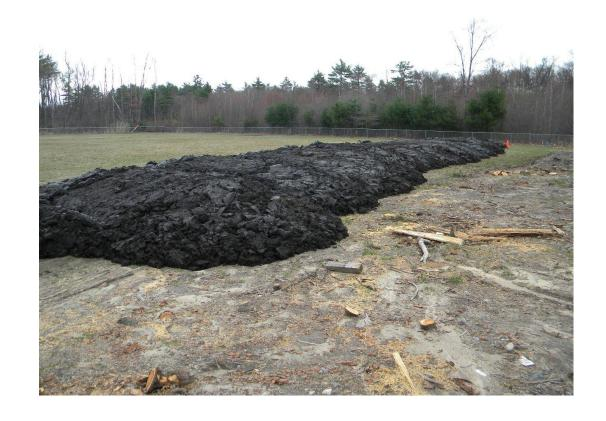
Reuse stockpile area with sediment being stacked higher to save space (intended reuse as ball field topsoil) – sediment now well dewatered
