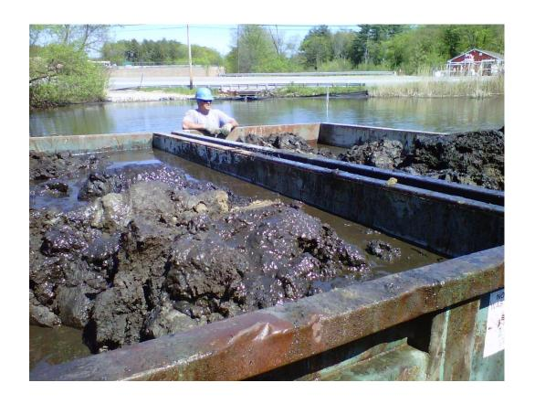
Contained clamshell dredged sediment dewatering area after overnight dewatering
