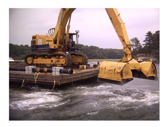
Standard excavator on sectional barge filling dumpsters – readily available, excavators known to fall off barges if not well chained down, can deal with debris including chain, moorings, stumps, logs, boulders, etc.; can be difficult to dig harder bottoms in deeper water due to barge movements
