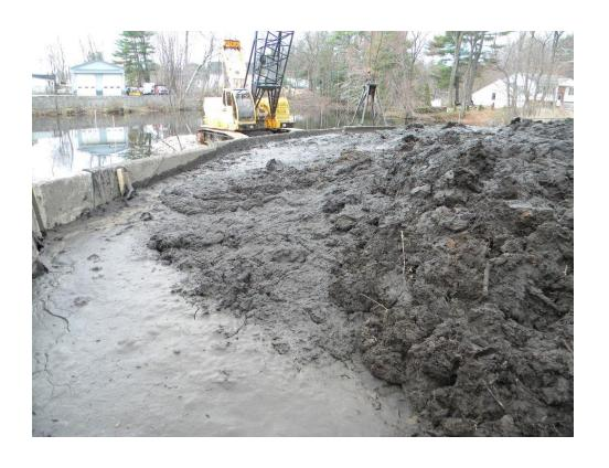
Same sediment being loaded for trucking with 1 to 2 day dewatering, EPA Paint Filter Test used as rapid onsite test by contractor to check for adequate dewatering for trucking with no seepage onto roads
