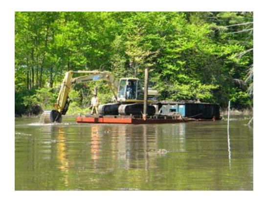
Mechanical dredging has an advantage in handling varying types densities of sediments with minimal addition of water or sediment bulking, aiding dewatering (hydraulic dredging entrains water to create a pumpable slurry which can take much longer to dewater, producing lower density fills that need soil densification on filled lands)
